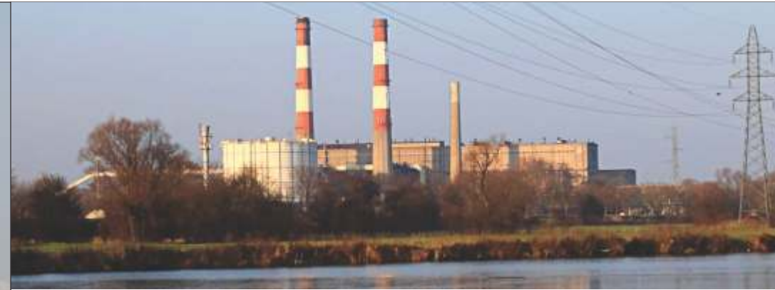
Power Plant, Koradi
