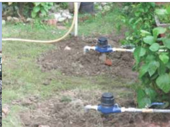
Rehabilitated House Service Connection
