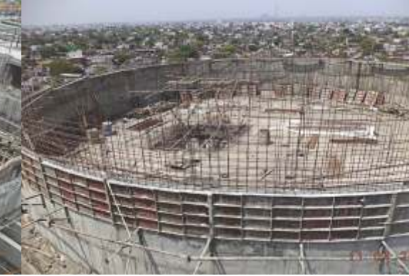
ESR Under Construction
