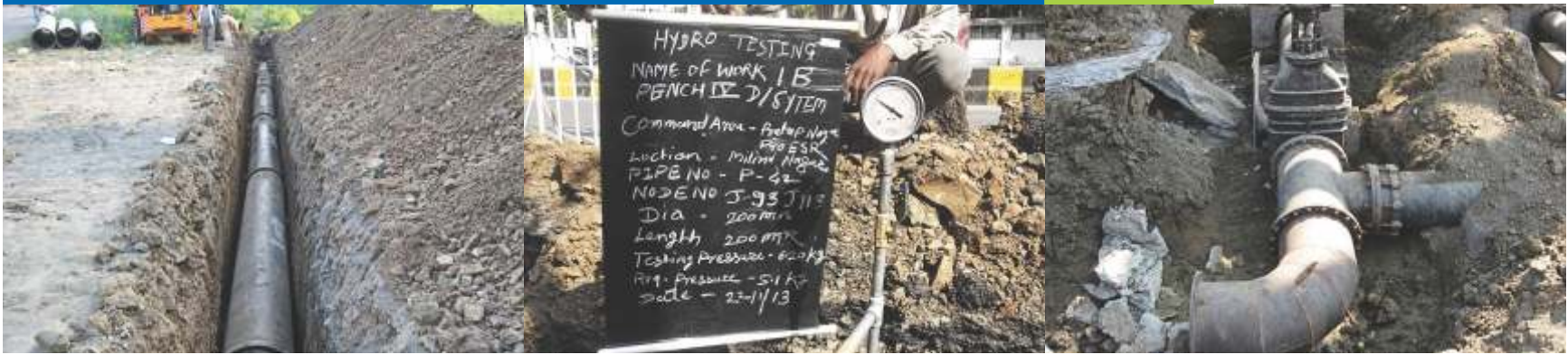
Distribution Pipe - DI Hydro Testing - Distribution Pipe Connecting ESR with Distribution
