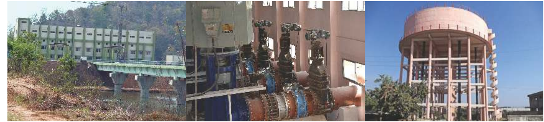
Pump house & Access Bridge
