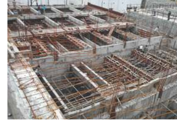
WTP 115mld Under Construction
