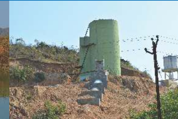
Break Pressure Tank
